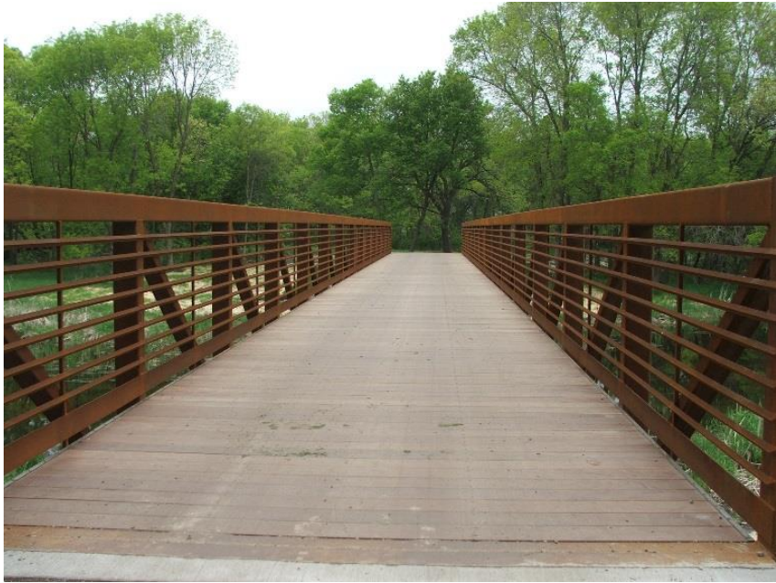
Pedestrian Bridge Example
