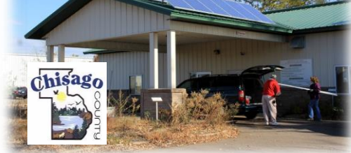
Staff unloading waste at the HHW Facility.
