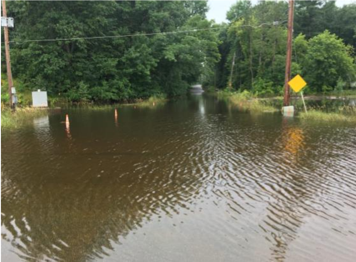
Entrance to Central Avenue neighborhood near Mora Lake, July 2018
