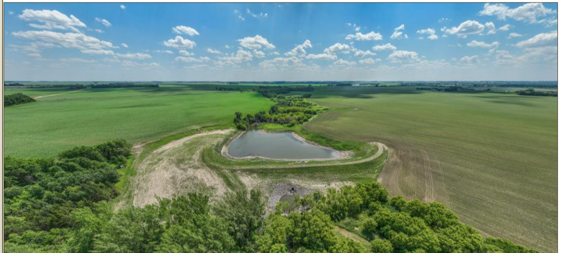
SPRINGDALE 19 GRADE STABILIZATION (Redwood County, 2021)
