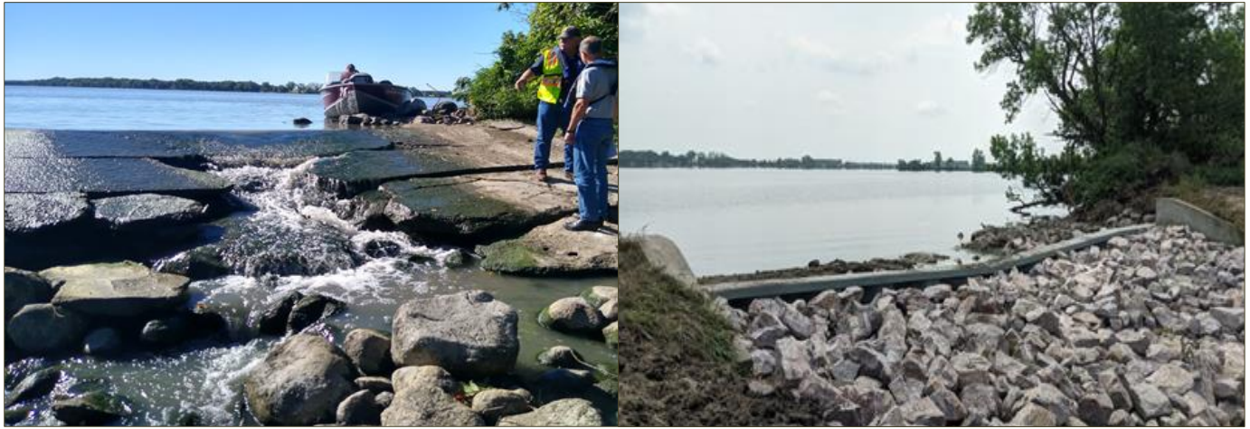
LAKE BENTON OUTLET RESTORATION (Lincoln County, 2021)
