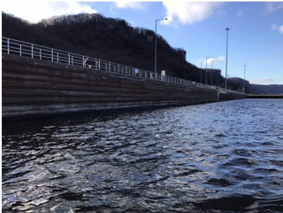
Figure 5 - Land Wall: Overall Good Condition
