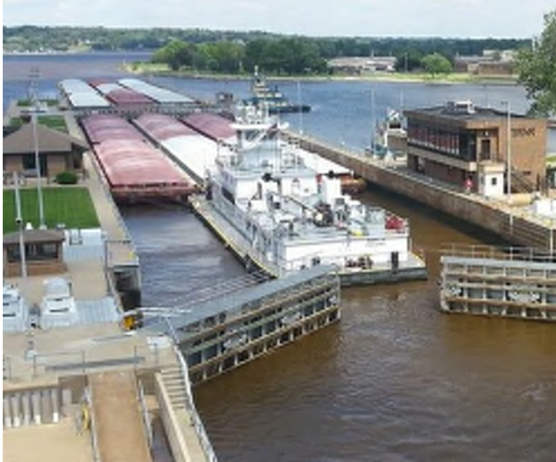
Figure 3 Example of a Lock
