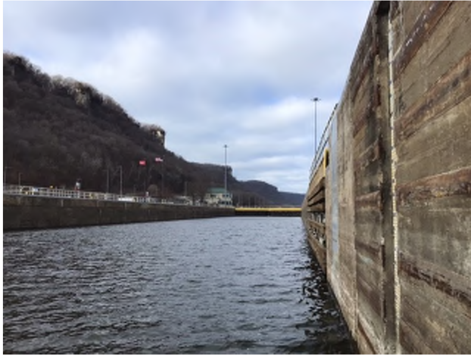
Figure 4 - I-Wall: Overall Good Condition
