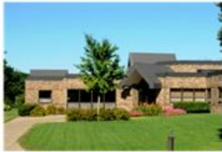
MCF-Shakopee built 1986 capacity: 656
