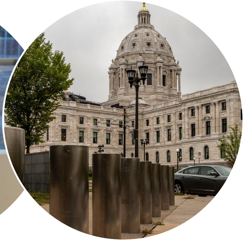
Capitol Complex Security Upgrades Phase II $33.4 million GO, $13 million GF
