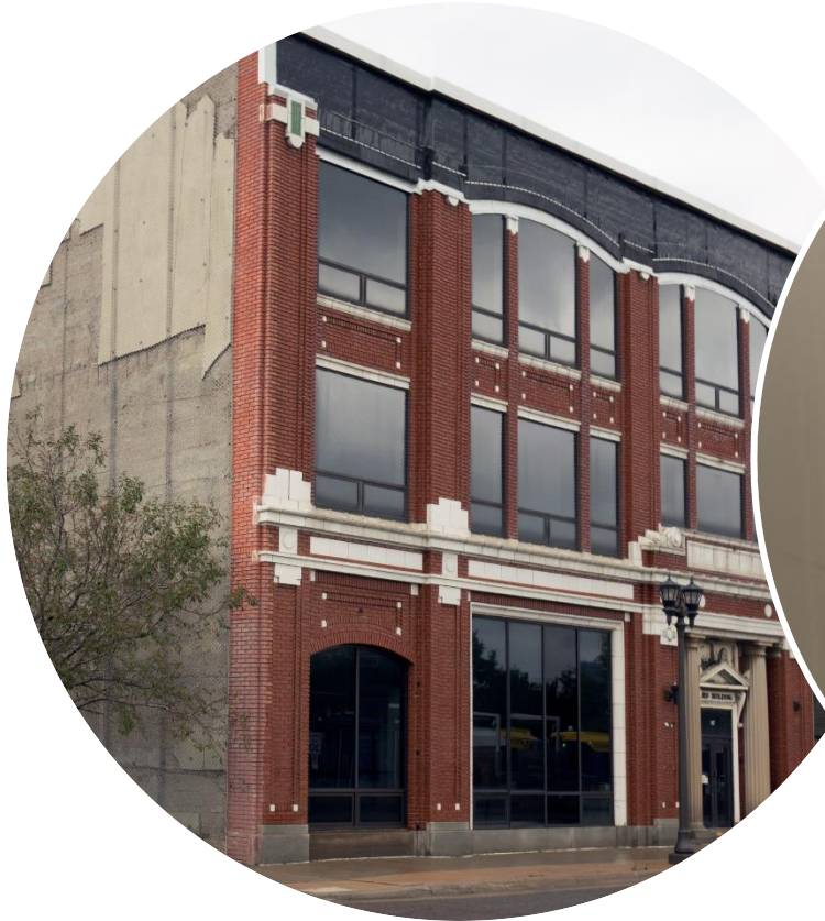
Ford Building Site 3.626 million GO
