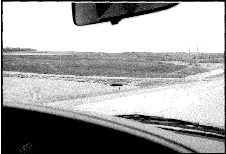
Rock Lake 15 Road Retention Lyon County
