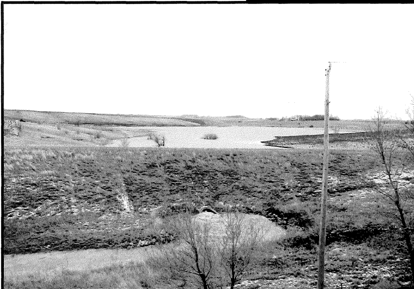
Rock Lake 21 Dam Lyon County
