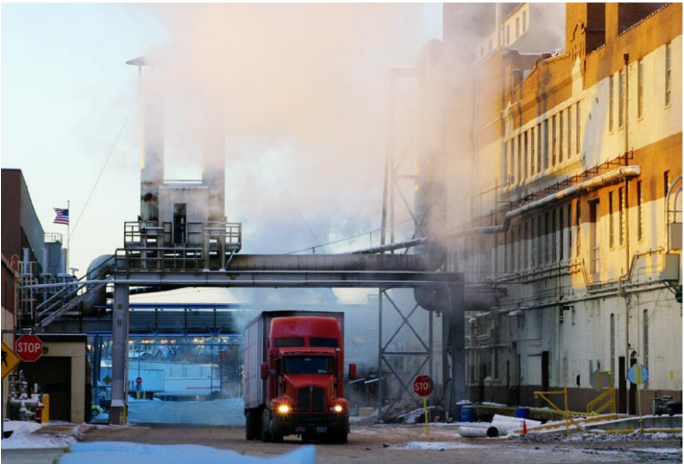
Rock Tenn paper processing plant in St. Paul.
