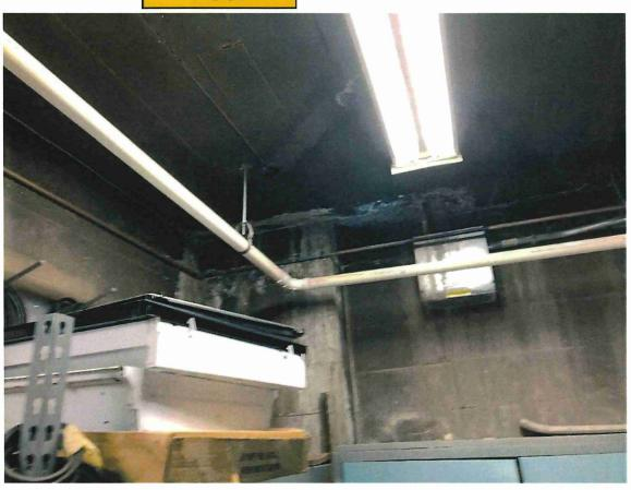
Age, Build-up in Waste Piping, Inadequate Slope for Low Flow Fixtures, Insufficient Valving
