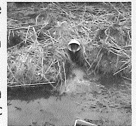
Drain pipe emptying into ditch
