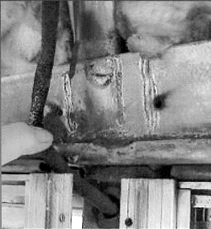
Cracked Weld (about ½ inch above wire grommet; wire held to side for visibility)
