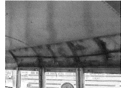
Light panel removed for inspection
