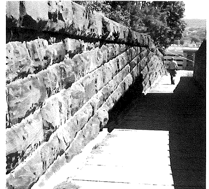
Walnut Street Retaining Wall
