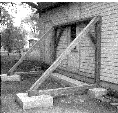
Ice House Temporary Stabilization
