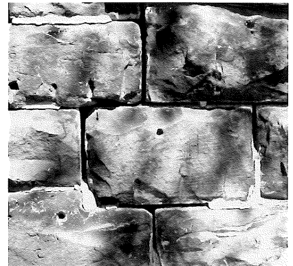
Walnut Street Retaining Wall
