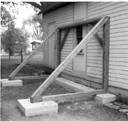
Ice House Temporary Stabilization
