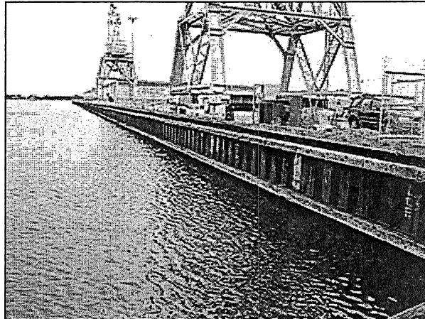
The Duluth Seaway Port Authority's bulk cargo dock is typical of many in the port. Steel sheeting, visible a few feet above the water line, drops vertically through 25 or 30 feet of water and another 20 into the harbor floor. The steel is up to one-half inch thick. (MPR Photo/Bob Kelleher)
