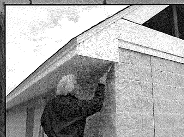
Restoration of building and facility maintenance.
