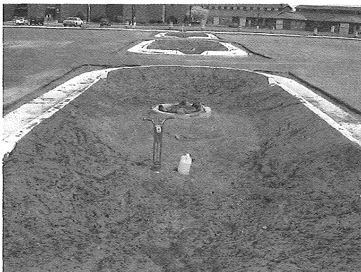
Figure 5. Rainwater garden composed of 70 percent sand, and 30 percent compost.
