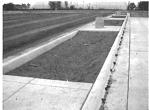
Figure 4. Structural soils are installed in a circle under the concrete pavement to the right and future bituminous surfacing to the left, about a 15-foot radius.
