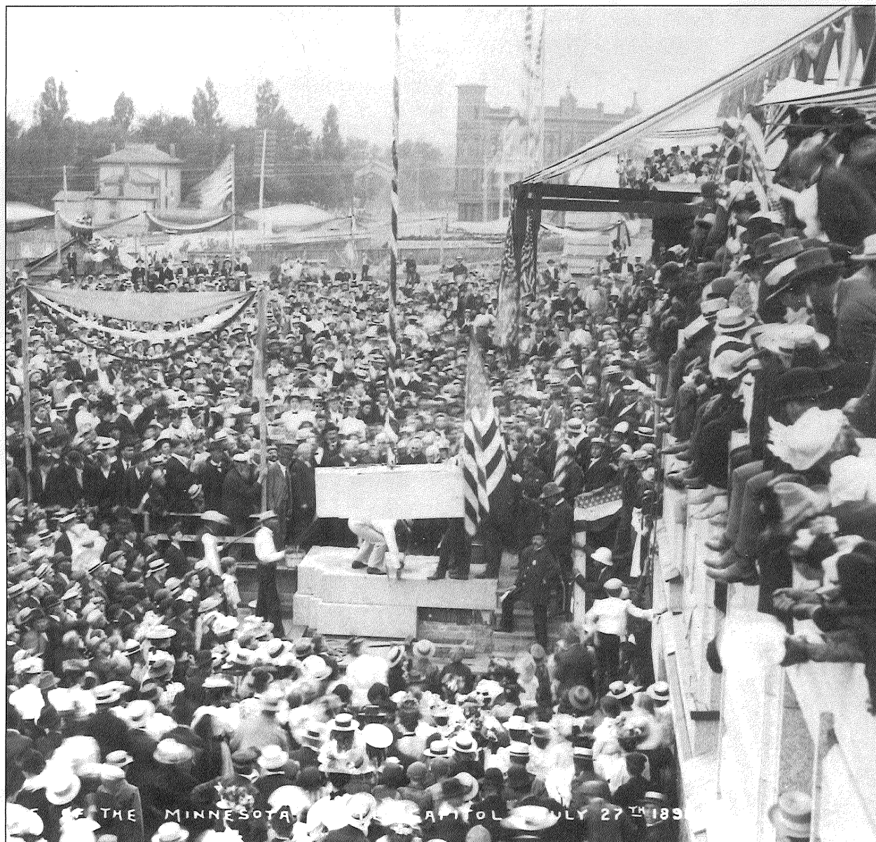
Laying the cornerstone for the new Capitol, July 27, 1898.
