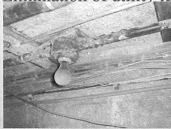
Deteriorating electrical system
