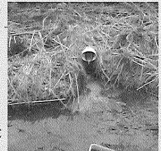
Drain pipe emptying into ditch
