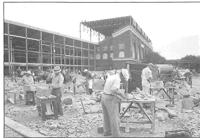
Works Progress Administration rock cutters prepare rock for a stone wall connecting the state fairgrounds’ race track.
